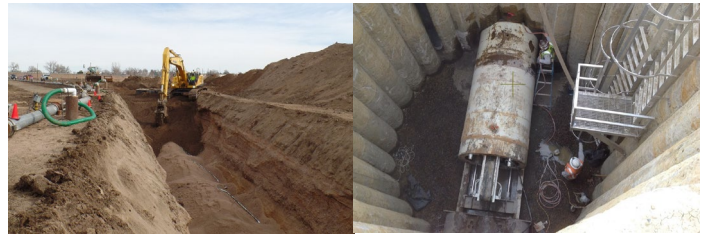
Examples of open-cut (left) and trenchless (right) construction similar to Second Creek Pipeline installation methods.
